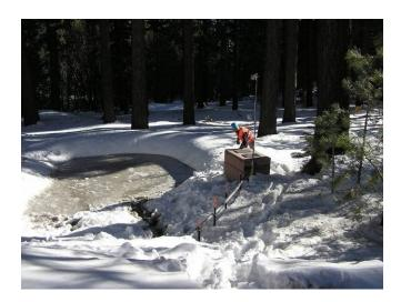
Figure A3. Looking southeast from corner of Harold Drive and Village Blvd., standing on the treatment vault. Water exits the vault and goes into a small detention basin (left). The equipment enclosure is being cleaned of snow (right). Photo courtesy of NTCD.
