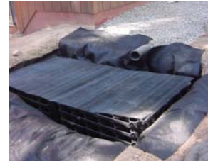
Rainstore with Geotextile
