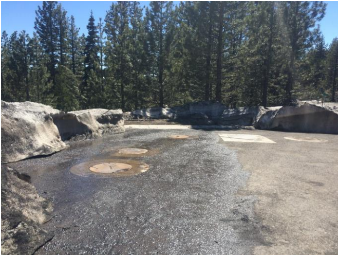
Figure 1: May 1, 2017, overland snowmelt flowing into CO manhole cover.
