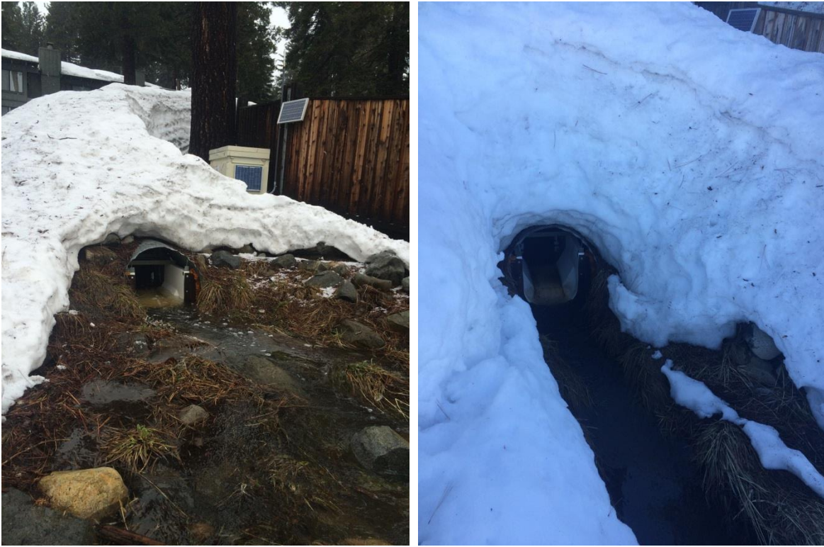
Figure 67 Staff worked hard to keep sites clear of snow during the very wet 2017 winter. Tahoma outfall pictured.
