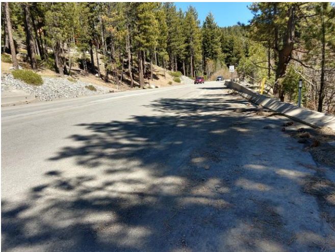
Figure 3: April 20, 2018 sediment on pullout and road.
