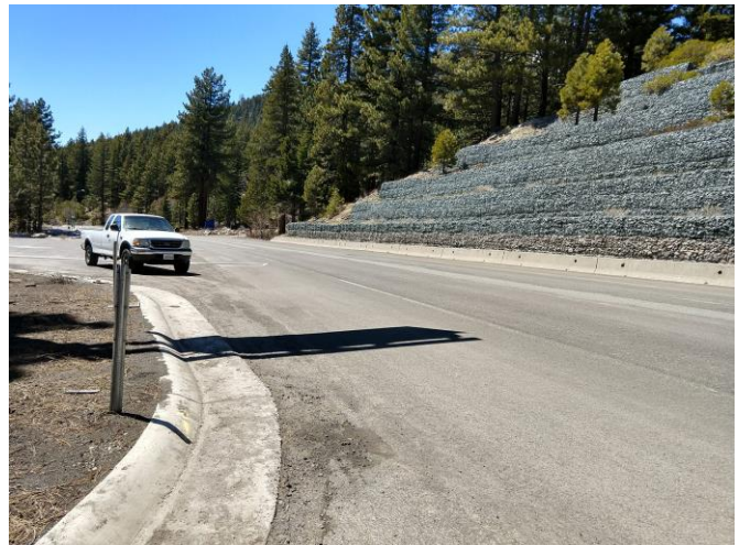
Figure 4: April 20, 2018 sediment on pullout and road.
