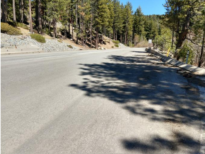
Figure 1: April 20, 2018 sediment on pullout and road.
