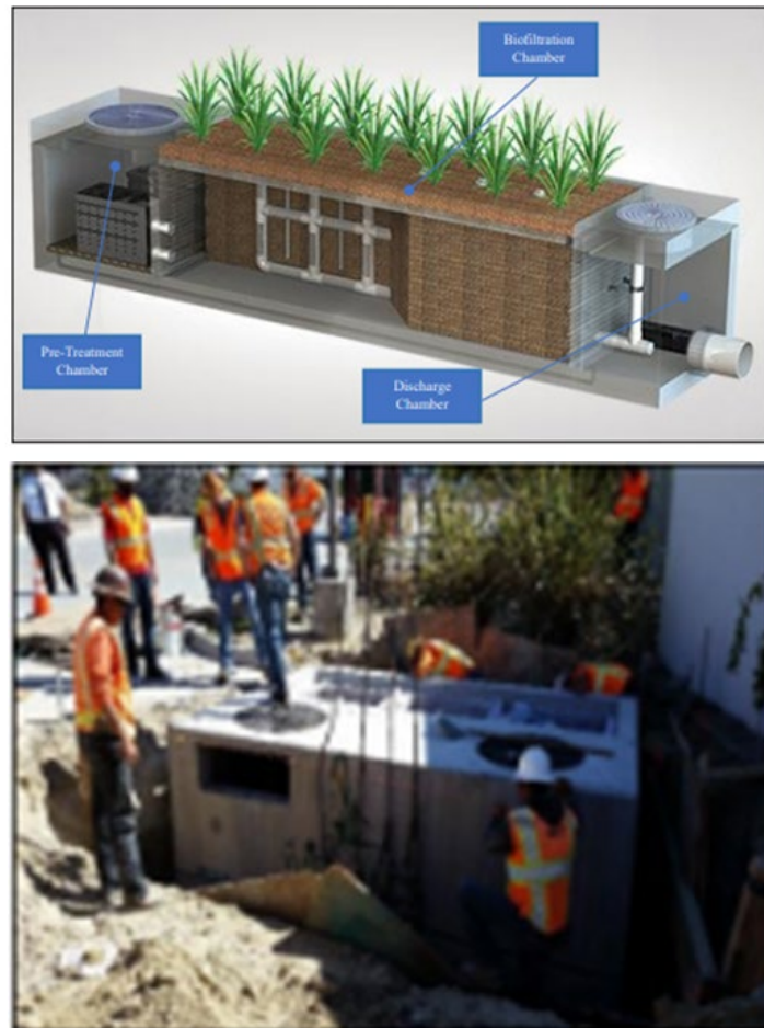
Figure A-6: Schematic of modular wetlands. Washington State TAPE https://ecology.wa.gov/ .
