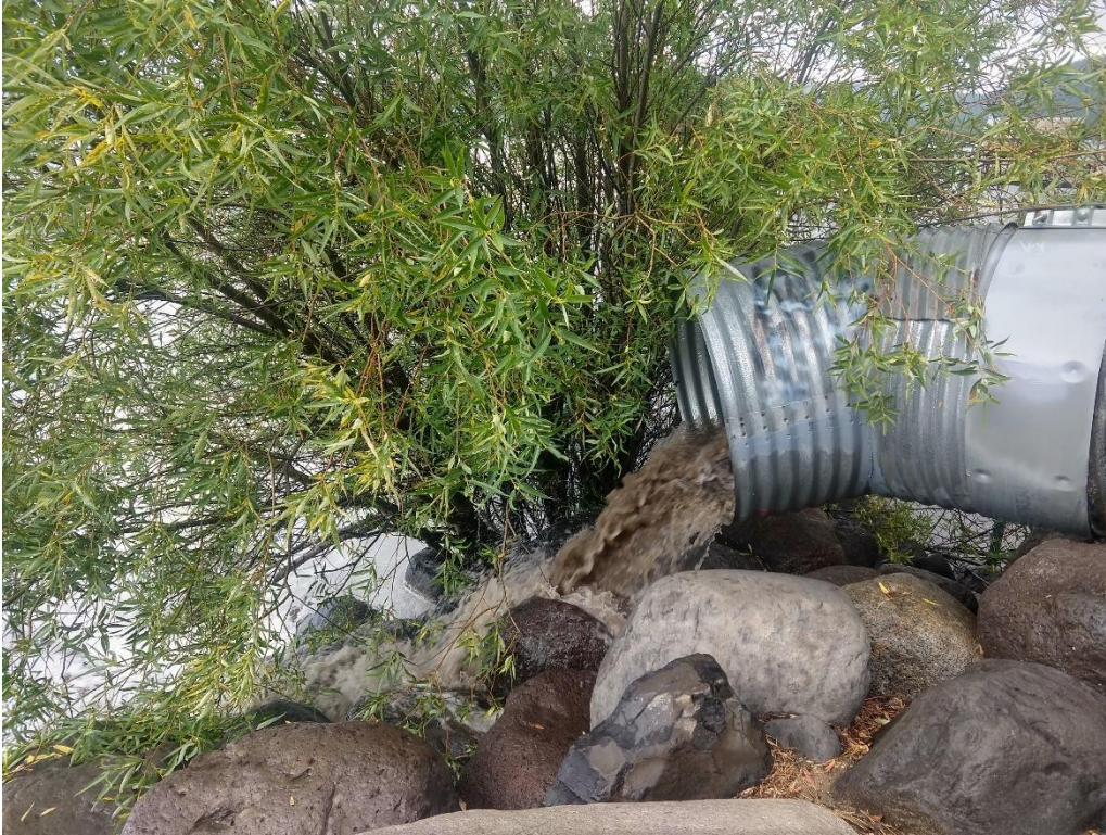
Figure 122 Flow during a thunderstorm event at Pasadena on July 16, 2020. Thunderstorm events can be difficult to monitor due to their short duration and episodic nature. Remote monitoring equipment makes sampling these events much more reliable.
