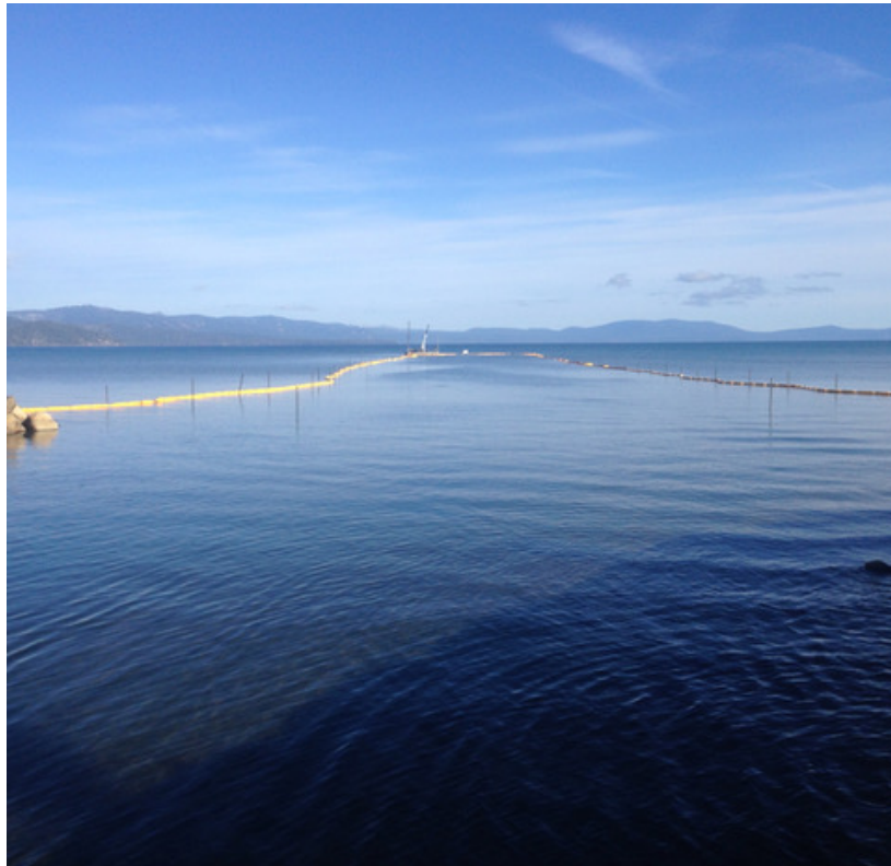
Silt curtain in Lake Tahoe to contain turbidity and nutrients
