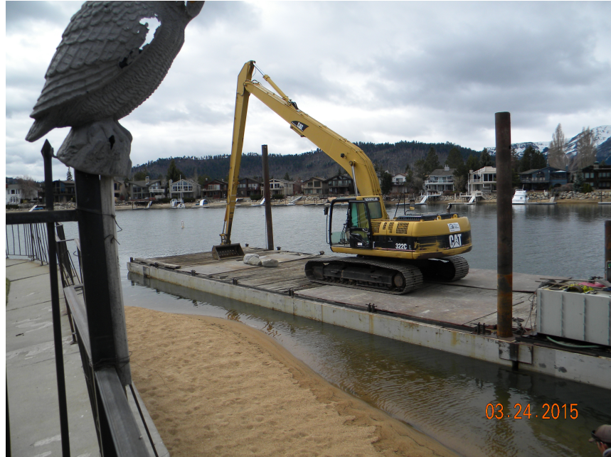
Mechanical dredging equipment at Tahoe Keys ( https://www.tkpoa.com/images/photos/projects/dredging/dredging5348.JPG )
