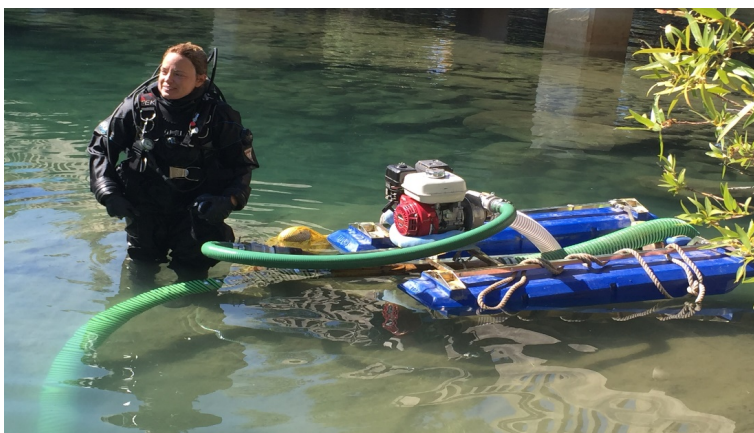
Diver with equipment on floating platform
