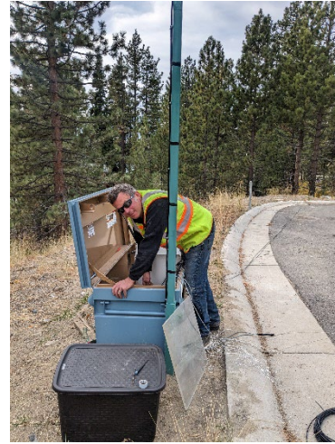
Figure 6 Reinstalling and troubleshooting equipment on November 1, 2023.
