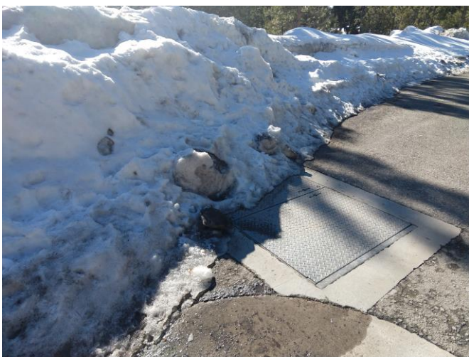
Figure 1: Berm on SR431 pullout after December 2019 storms. This berm made it impossible to access sites.
