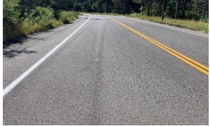
Figure 74 Elks Club Drive after repaving. (A Buxton)
