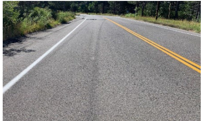
Figure 74 Elks Club Drive after repaving. (A Buxton)
