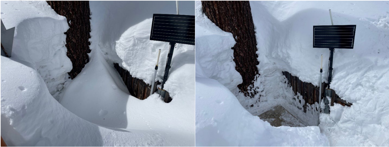
Figure 135 Snow at Tahoma March 7, 2023 before snow removal (image 1) and after snow removal (image 2). It is critical to stay on top of snow removal after snowfall events to maintain access to stormwater monitoring sites.
