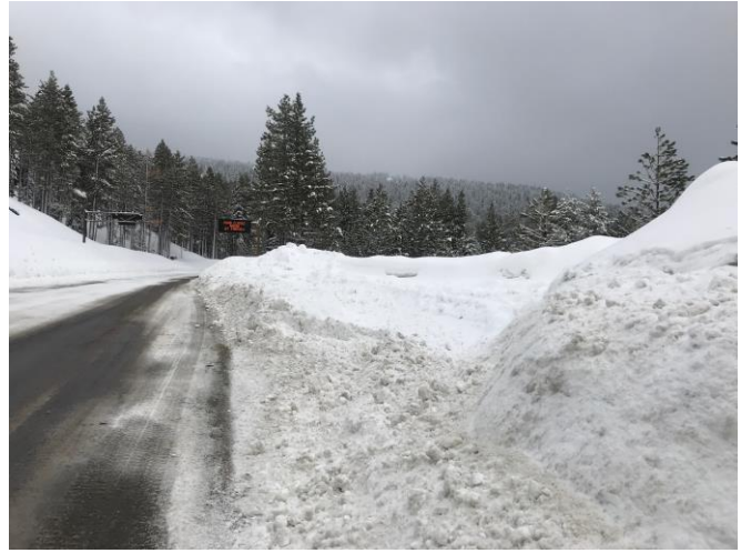
Figure 4: February 28, 2019 berm on road. Access doors are under several feet of snow in the pullout.
