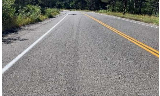
Figure 74 Elks Club Drive after repaving. (A Buxton)
