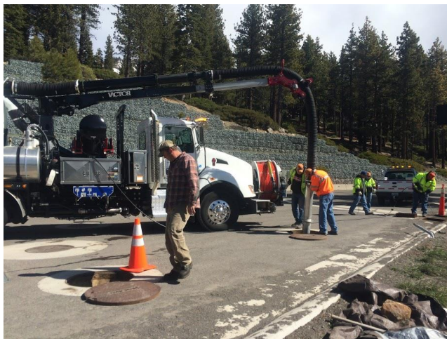
Vector truck cleanout on 4/15/16 at SR431 (left). Note accumulated sediment along the curb. Sediment filled flume prior to cleanout (right).
