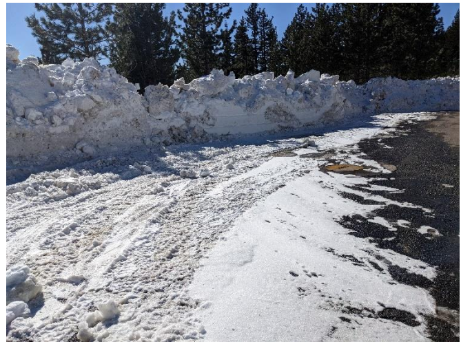
Figure 4 Berm at SR431 pullout on January 31, 2023.
