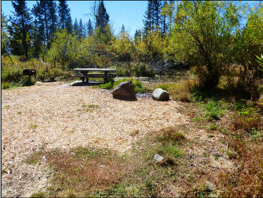
High water encroachment of a campsite. Photo date 10-5-18.
