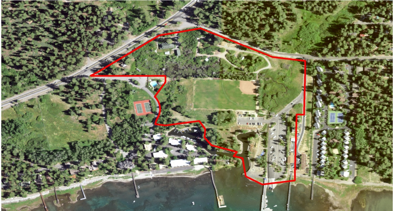
Figure 16. Aerial photograph from 2016 (Study Area outlined in red). The road connecting the campground to the boat ramp was removed and Lake Forest Creek realigned to a more natural planform. Improvements to the boat ramp and Pomin Park were also completed.
