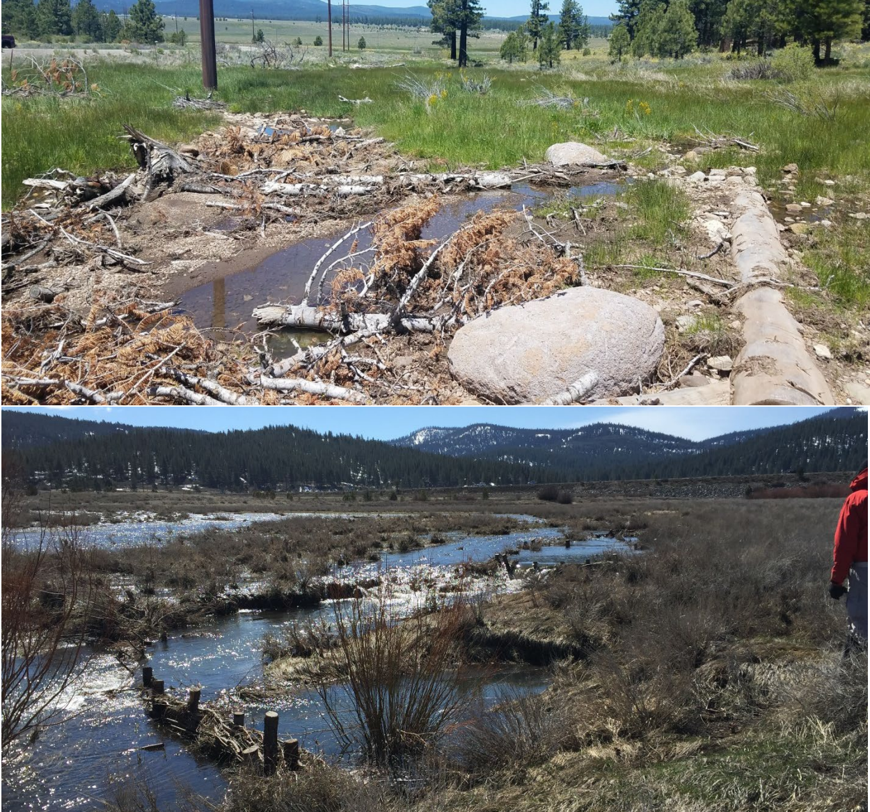
Figure 19. Examples of bio-engineered log structure (top) and debris jam (bottom). Both photos are taken from restoration projects constructed in Martis Valley (about 8 miles north of the Project Site) less than two years after construction and vegetation has not fully reestablished.
