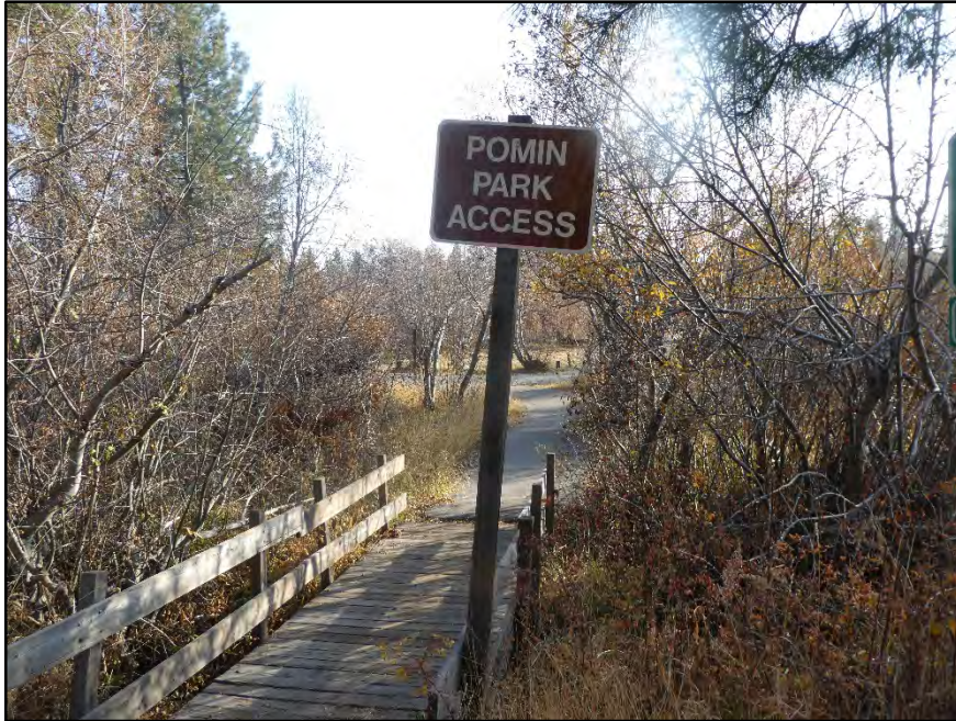
Bridge over drainage near Pomin Park entrance. Photo date 11-17-18.
