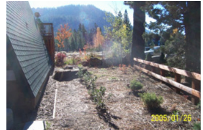
Post removal; revegetation
