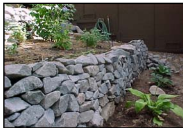
Rock Retaining Wall
