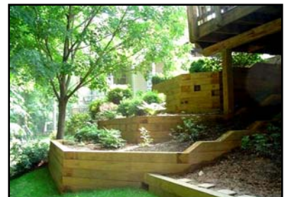
Wood Retaining Walls
