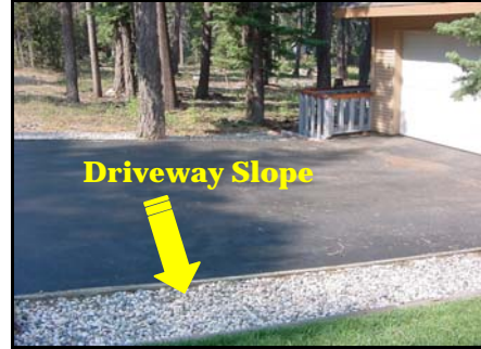
The runoff from the driveway above flows into the infiltration trench along the driveway edge.
